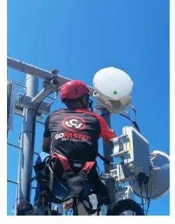
positively influenced the decision. After swapping out units to resolve a minor issue with using the SFP port, the installation proceeded as expected and was completed in less than one week. The small form factor antenna and Siklu's alignment tools also help to speed the deployment process.
