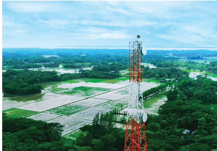
The 75-metre tower consists of an in-built green hybrid energy solution with a capacity to produce 42 kilowatts per day from 12-kilowatt solar panels and six kilowatt per day from four kilowatt wind turbines mounted on the tower
