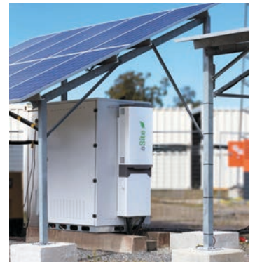
The eSite x10 is claimed to be the world's first hybrid power system purpose-built for outdoor telecom sites.
