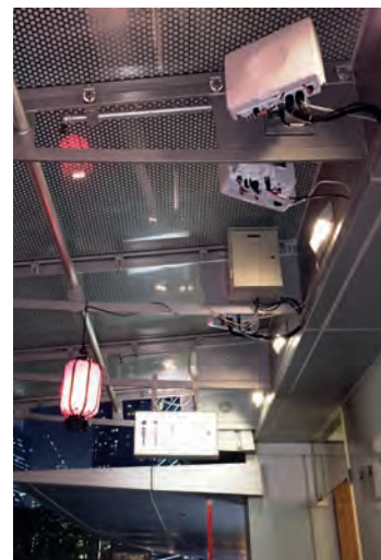
Nokia Networks' Flexi Zone small cells installed along the Marina Bay waterfront in Singapore.
