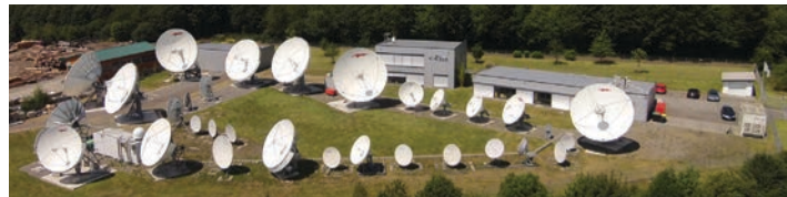
CETel's German teleport near Cologne and Bonn. The company says its antennas for standard C-band, extended C-band and Ku-band directly support geo-stationary and inclined satellites between 68°W and 75°E.
