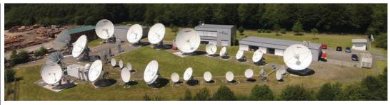
CETel's German teleport near Cologne and Bonn. The company says its antennas for standard C-band, extended C-band and Ku-band directly support geo-stationary and inclined satellites between 68°W and 75°E.
