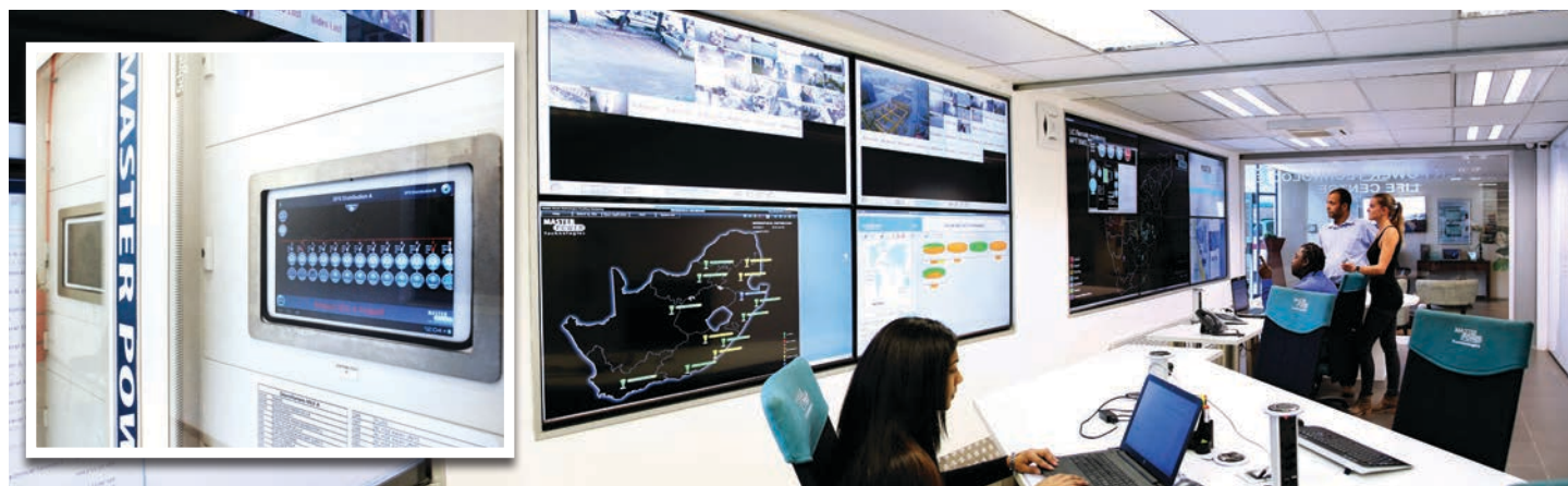
Main photo: MPT's NewLife Centre in South Africa monitors all secure power critical equipment for its customers in real-time. Inset: data from the company's intelligent Universal Controller can be accessed and displayed on touchscreens mounted in strategic locations.
