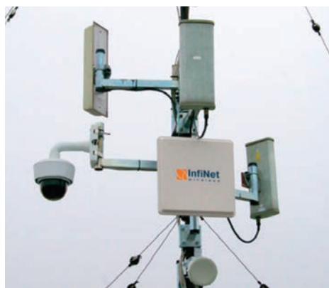
InfiNet Wireless' InfiLINK 2x2 wireless infrastructure carries traffic from the IP cameras to the main operating centre in Cairo.
