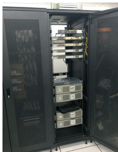
Carrier-grade switching and termination equipment used to power VAST's Wi-Fi network. The firm says it continually investigates a variety of technologies, such as DAS, LTE-U, LAA and LWA.
