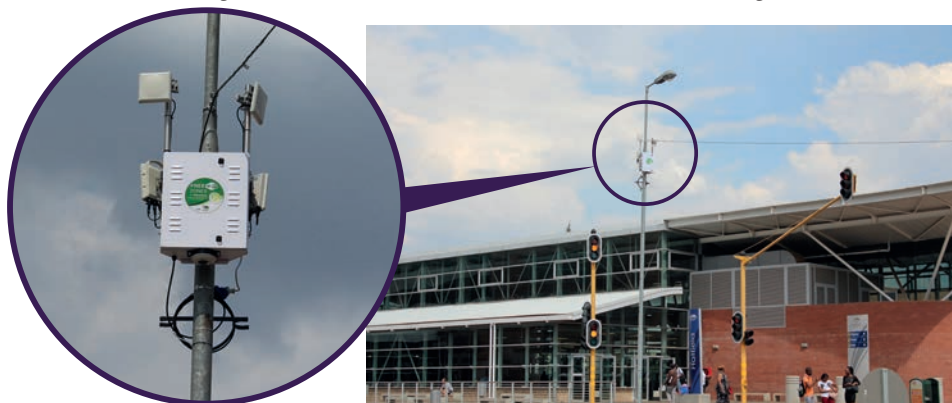
RADWIN's base stations provide continuous coverage and broadband connectivity to the buses in motion. The stations deliver up to 100Mbps but can go up to 250Mbps in MIMO mode.
