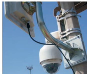
Installing a line-of-sight video surveillance system at the Port of Dakar's four container terminals proved challenging as 16 metres was the maximum height available for camera locations.
