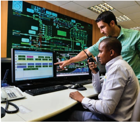
Teltronic's CeCo-TRANS system is used by control centre operators at Nacala Port in Mozambique. The TETRA app displays train fleet positions in real-time.
