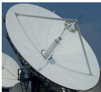
Arabsat and CETel have built an Earth station which uses a 9.3m antenna at CETel's teleport in Germany.
